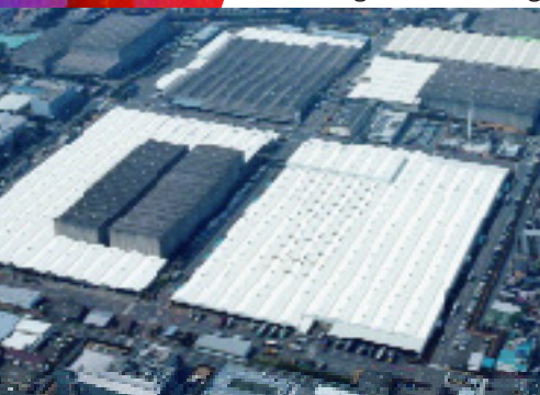
Nissan Building—After coating
